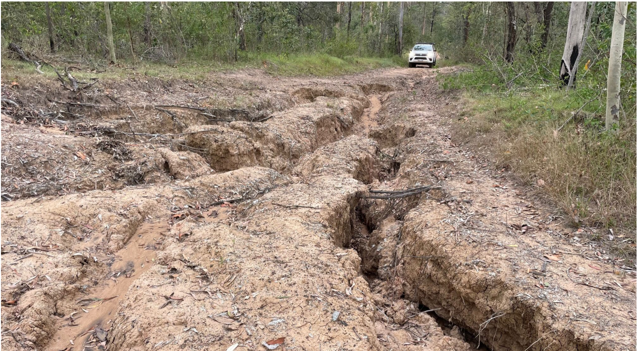
Photograph 4: Unsealed track in western parts of Precinct A displaying signs of significant erosion.
