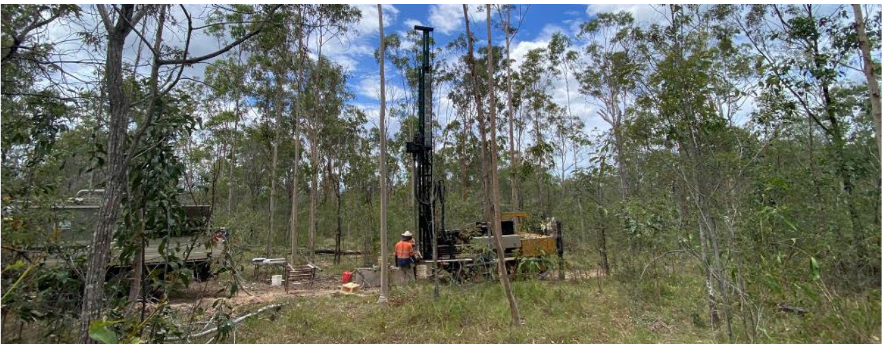
Photograph 3: General site conditions (view looking towards borehole BH4)
