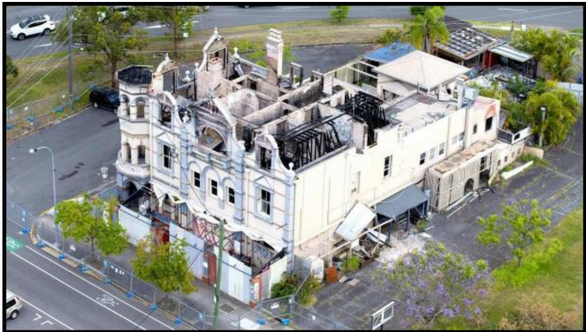
Figure 2.3.2 The State Heritage Listed Broadway Hotel (imagery date: 2021)
