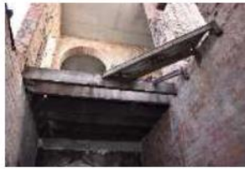
Figure A2.10 Stairwell GST
