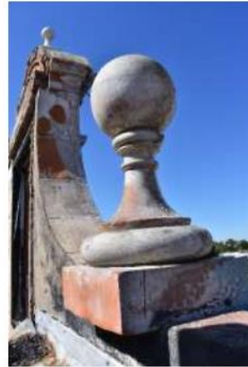
Figure A2.14 Terracotta parapet detail
