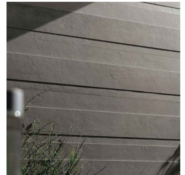
HORIZONTAL WALL BANDING
