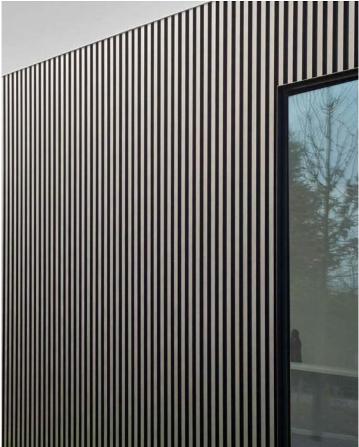
ALUMINIUM CLAD WALLS SEPARATING ADJACENT APARTMENT BALCONIES - NEUTRAL COLOUR
