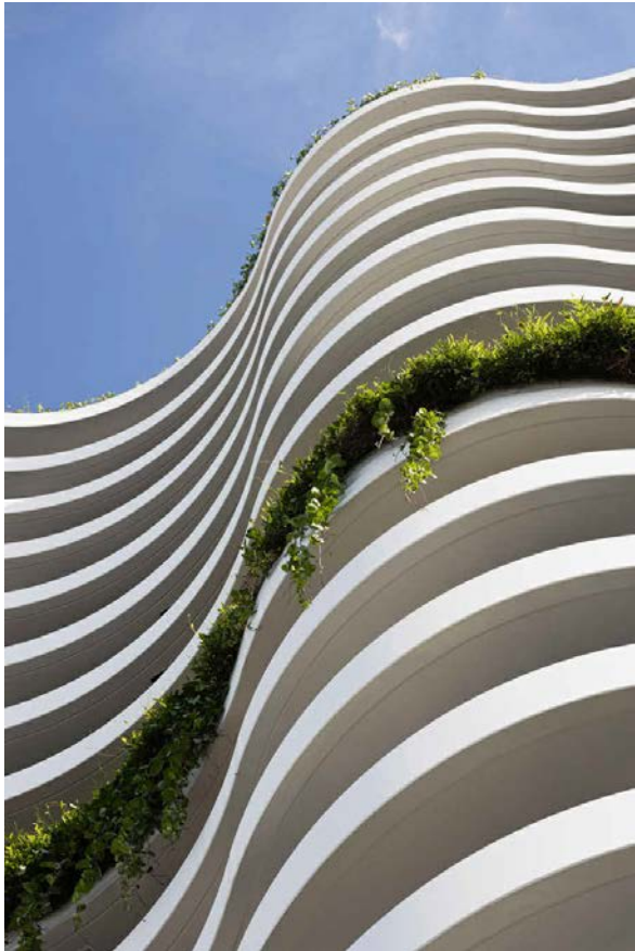
HANGING PLANTERS THROUGHOUT BUILDING
