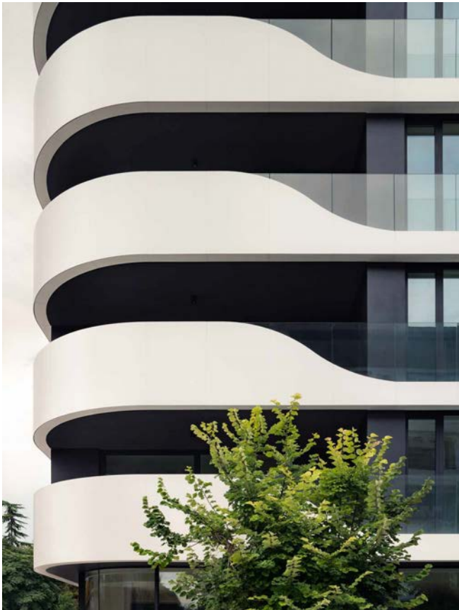
CONCRETE BALCONY WALLS CURVED AND STRAIGHT WALLS - PAINT FINISH
