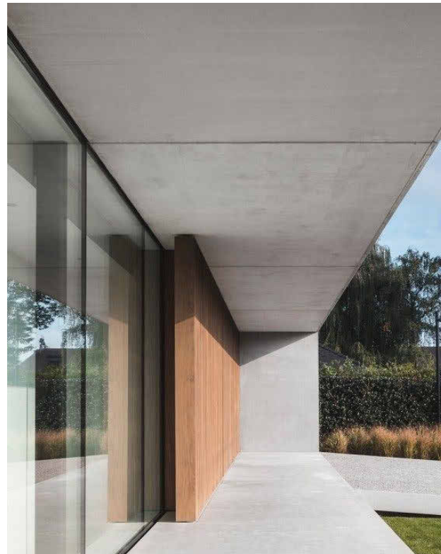
EXPOSED CONCRETE FLOORS AND WALLS
