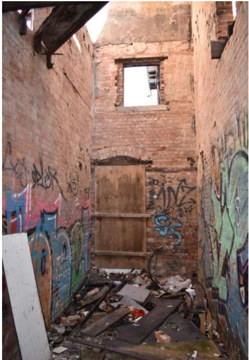
Figure 9 Ground floor stairwell in 2022
