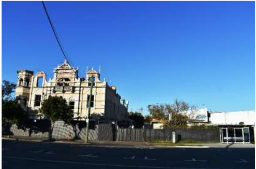
Figure A2.2 Logan Road frontage to site
