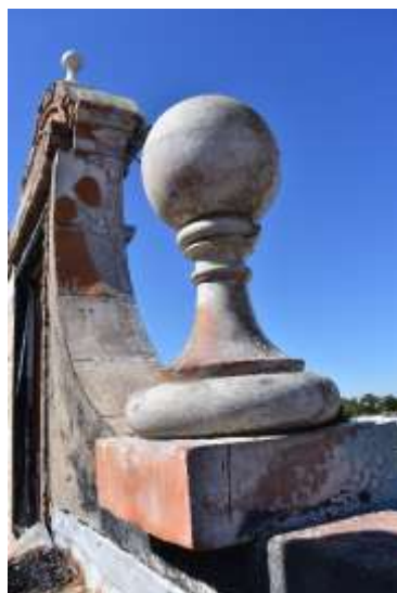
Figure A2.14 Terracotta parapet detail
