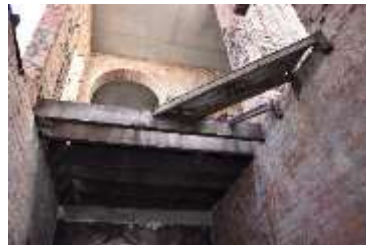
Figure A2.10 Stairwell GST
