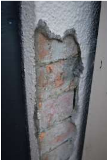
Figure A2.7 Rendered brickwork
