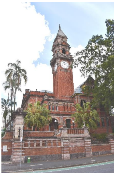
Figure 113 South Brisbane Town Hall
