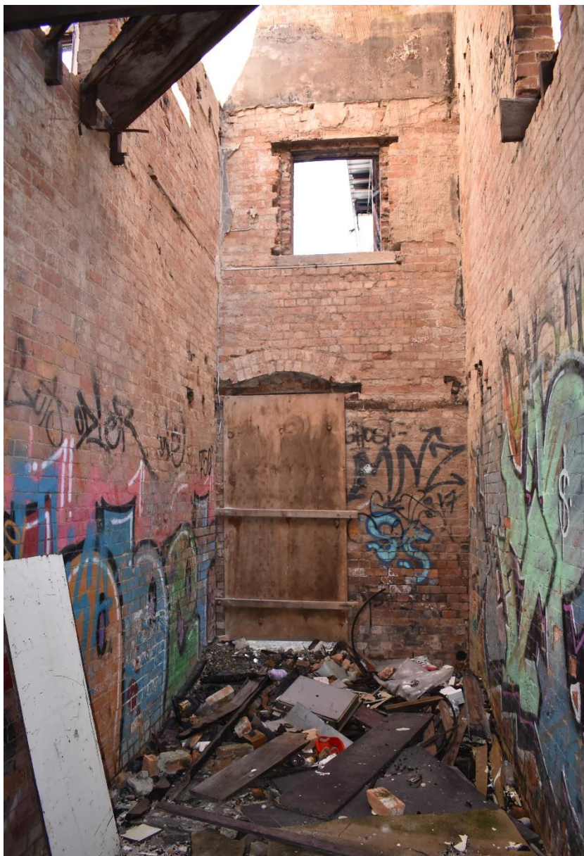
Figure 34 Ground floor stairwell in 2022
