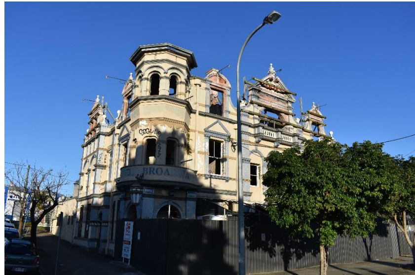
Figure 105 The Broadway Hotel's prominent corner turret
