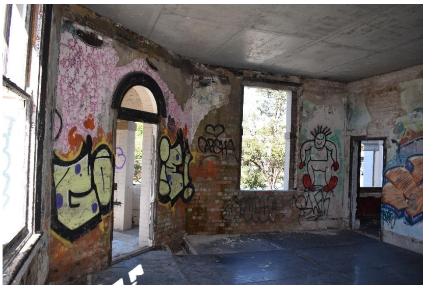
Figure 32 First floor corner room in 2022. Note the recent suspended concrete second floor slab above.
