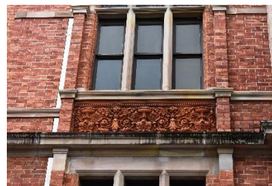
Figure 115 South Brisbane Town Hall
