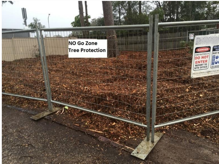
Figure 18: Standard TPF with ground protection mulch
