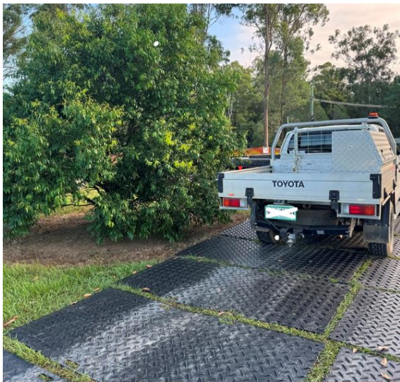
Figure 21: Light vehicle ground protection
