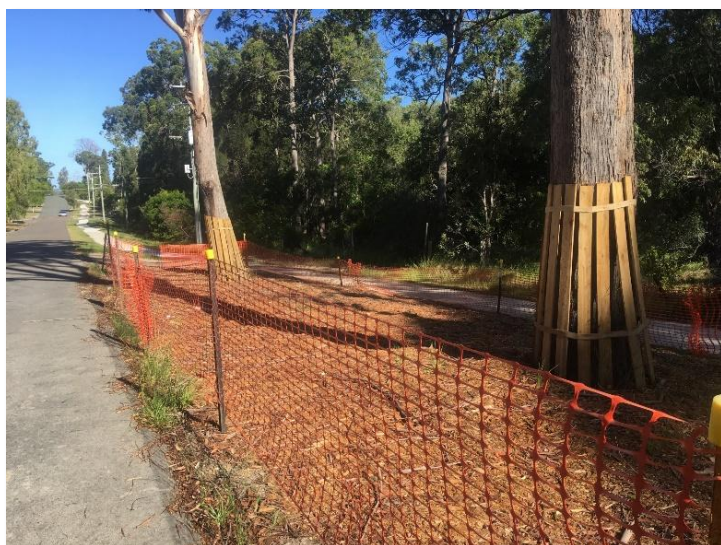
Figure 20: Exclusion Zones with Trunk Protection
