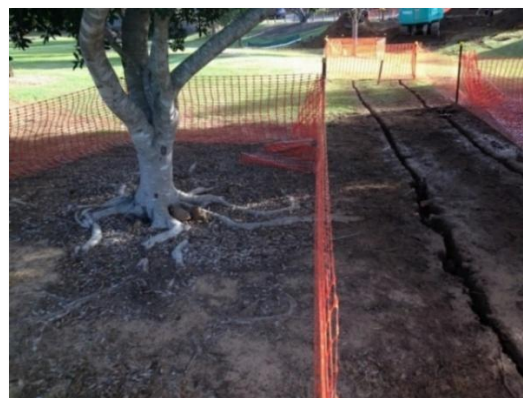
Figure 23: Example of preliminary trench/excavation cuts
