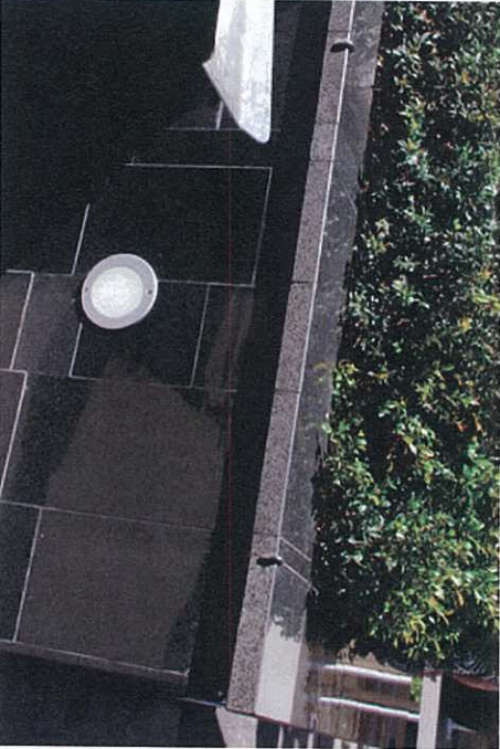
Raised planters finished to match existing Portside detail
