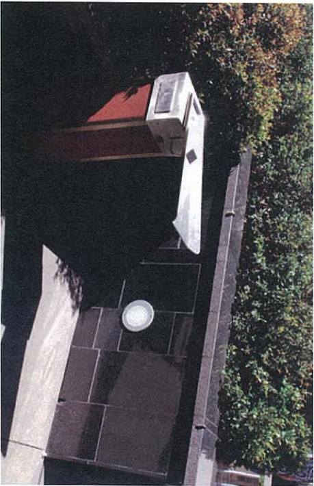
Paving and ground surface treatments wrapping up podium walls providing a continuation and integration of materials
