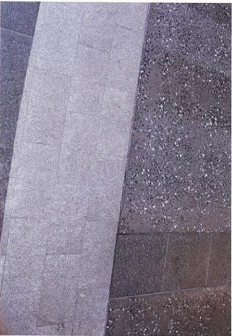
Paving differentiation to define pedestrian and vehicular zones and assist with way finding
