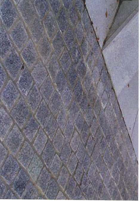
Small format pavers to laneway to highlight change of environment and bring intimate scale to the space
