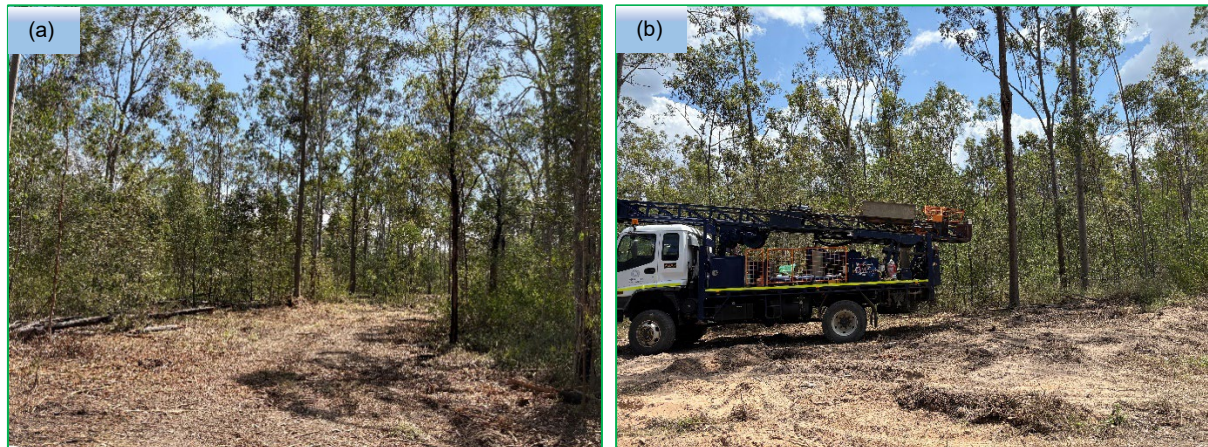
Figure 4: Photographs Showing the General Site Conditions
