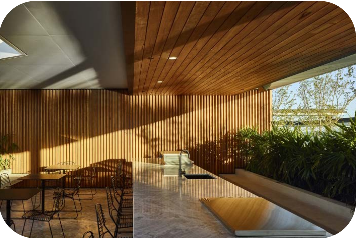
Timber roof & batten panelling
