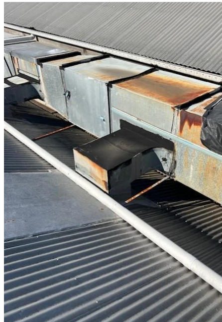
Figure 29: Existing ductwork on roof
