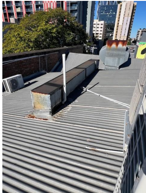
Figure 31: Existing ductwork on roof
