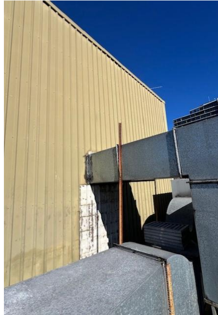
Figure 27: Existing ductwork on roof
