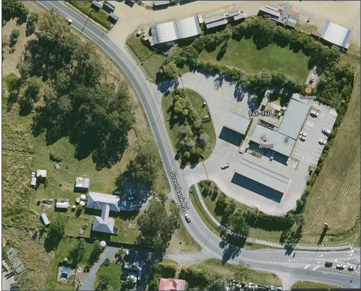
Figure 2.3 Existing Ampol Service Station
