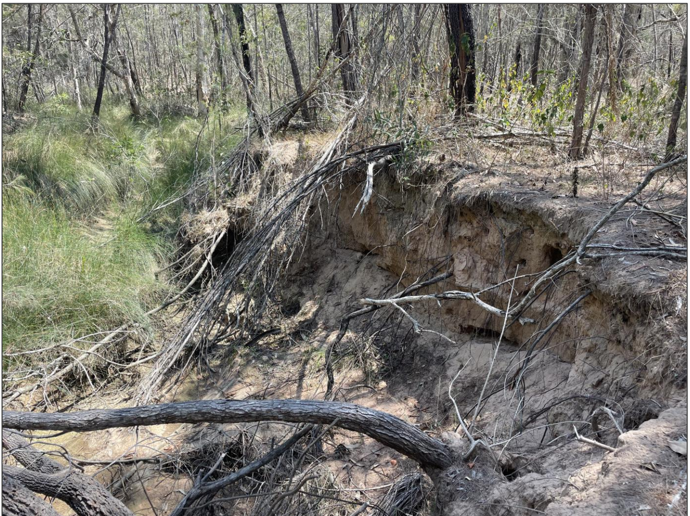
Figure 4.1: Existing Eroded Creek Line within the Site
