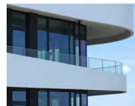
06 GLASS BALUSTRADE COLOUR DARK GREY HANDRAIL
