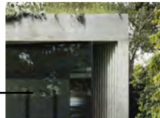
03 OFF FORM CONCRETE COLOUR CONCRETE FINISH
