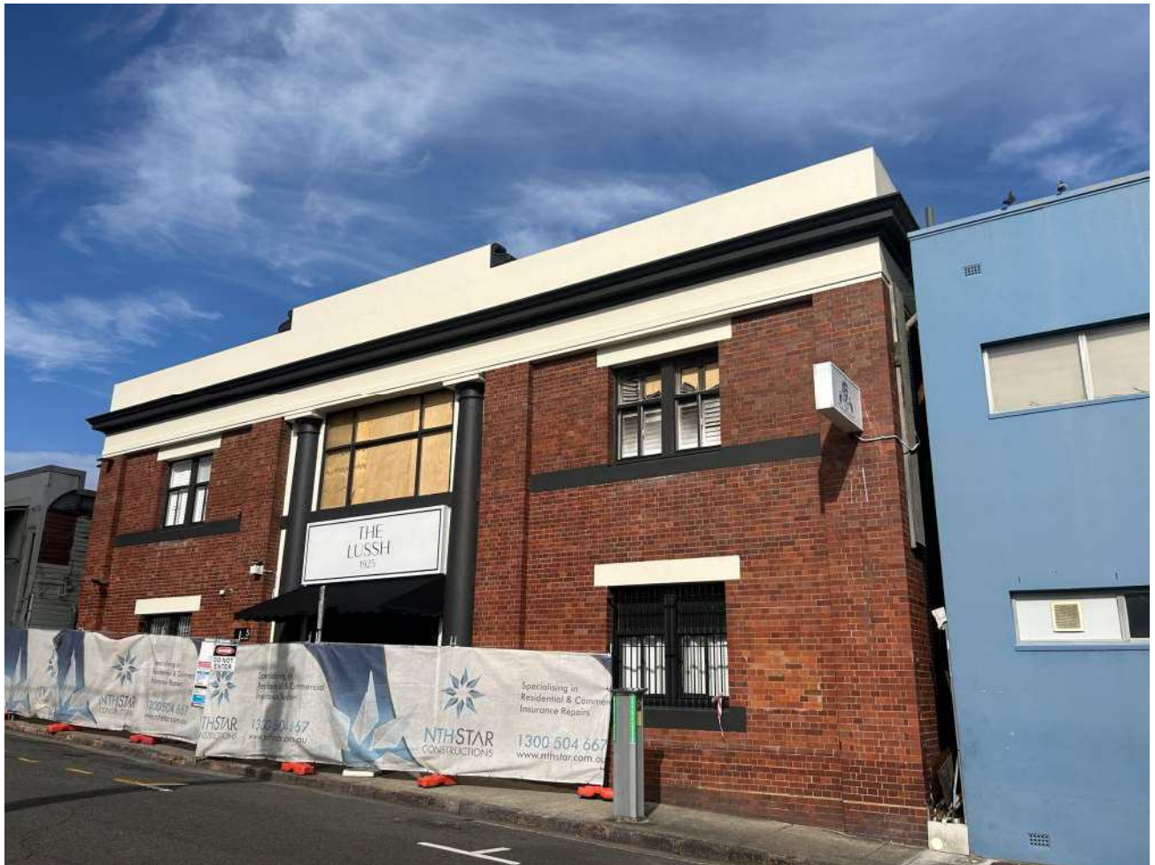
Figure 14 – Hubert Street Front Building Façade, Structurally Undamaged from the Fire Event.
