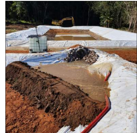
DEWATER LOW LYING AREAS BY PUMPING TO HES BASIN
