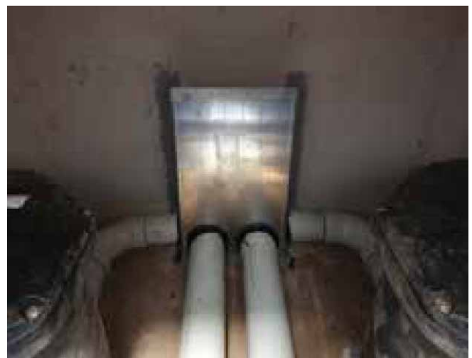
Figure 3 - Typical Outlet Weir Wall
