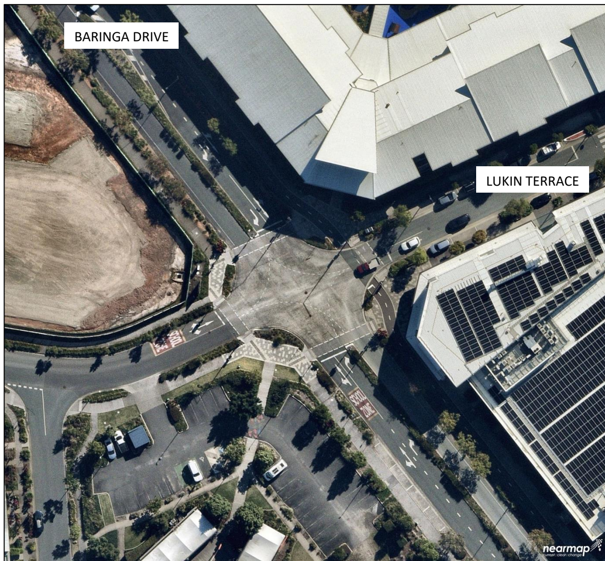
FIGURE 3.1 – AERIAL OF THE BARINGA DRIVE / LUKIN TERRACE INTERSECTION
