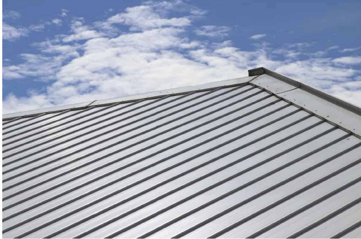
4. PROFILED METAL ROOFING
