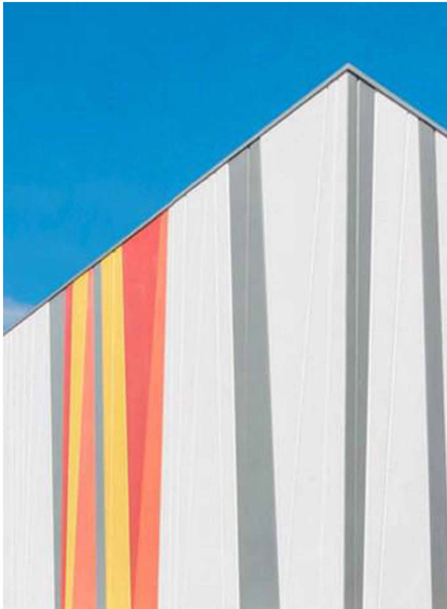
7. PAINT FINISH CONCRETE TILT-UP PANELS
