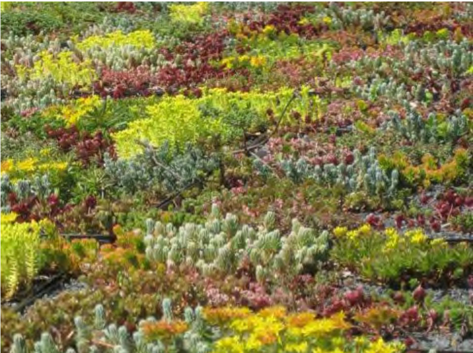
Exemplar rooftop planting
