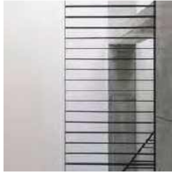
BALUSTRADE - PROTECTIVE COATING
