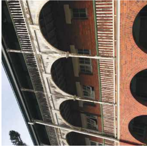
BALUSTRADA TYPE 1 - TIMBER
