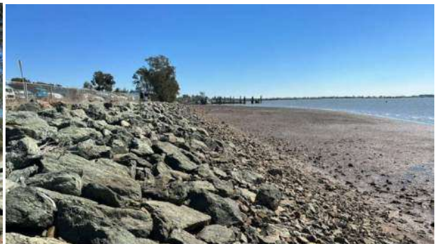
Photo 2 Southern medium deck location
