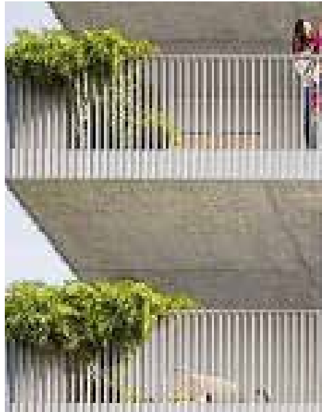
Neutral Coloured Painted Metal Balustrade for Walkways
