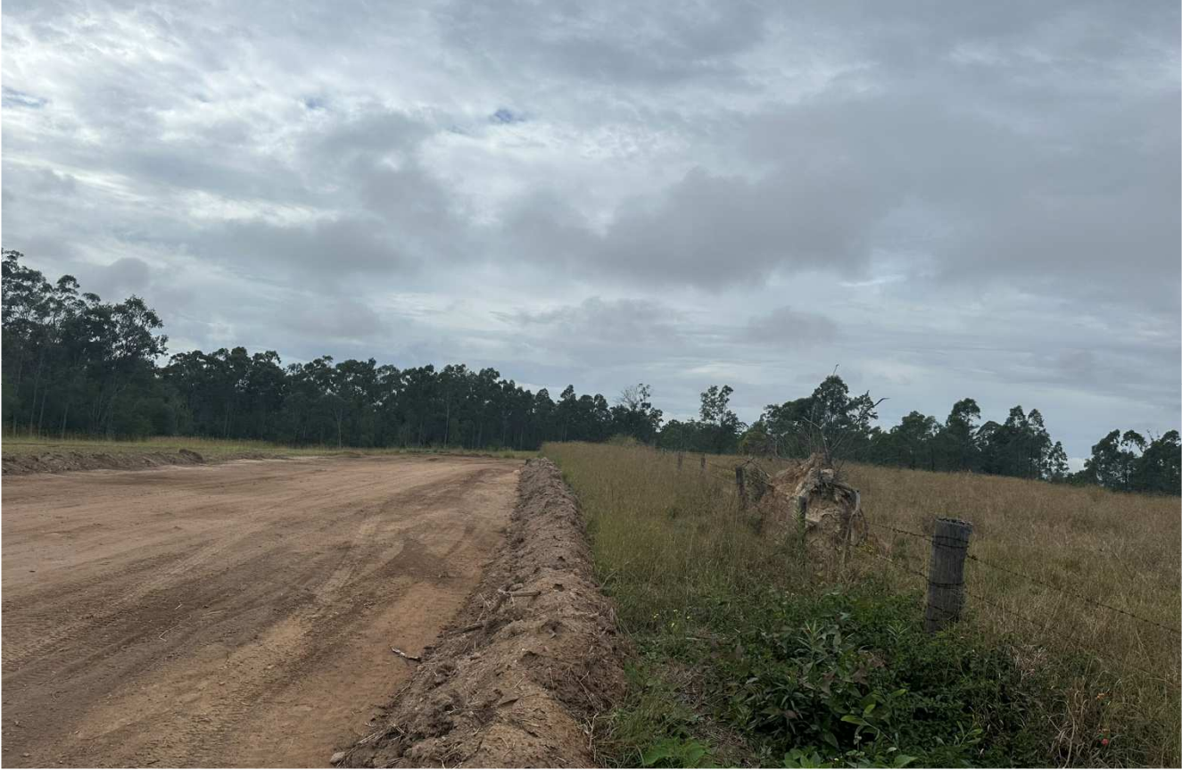
Photograph 3: Northeast corner of subject site (Source: SHG)
