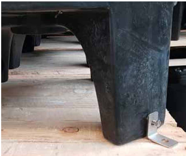
Figure 4 - Bolting the feet.
