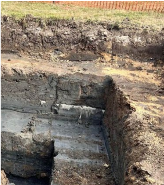
Image 8: Soil strata from surface to 3m BGL.
