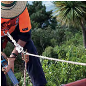
7 MAINTENANCE SAFETY Balcony planter and roof top planter maintenance must utilise 'anchor and harness' style fall protection systems (XSPplatforms 'LinkdPro' or like product)
