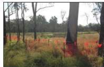
SIGNIFICANT TREE PROTECTION FENCING
