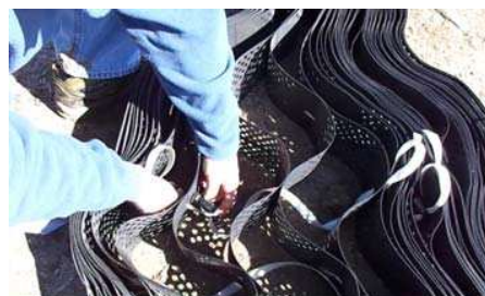
Figure 17 Threading Tendon and Attaching ATRA Tendon Clips
