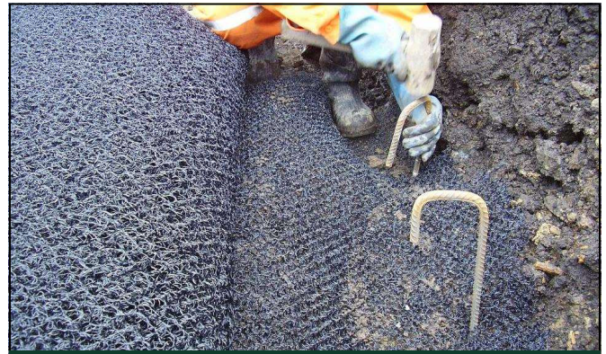
Fixing MacMat in trench
