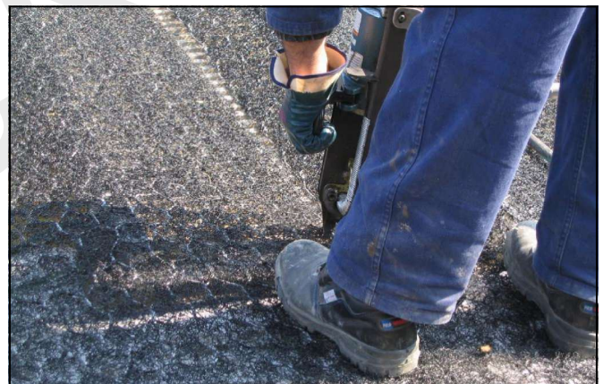
Connecting adjacent panels of MacMat® R with 'hog-rings'
