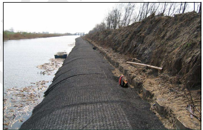
MacMat® R erosion protection on river bank
