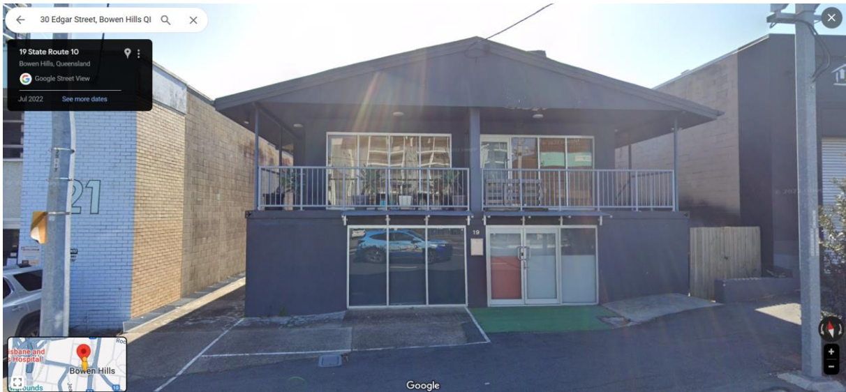
Figure 2-11 19 Campbell Street, Bowen Hills Source: Google Maps
