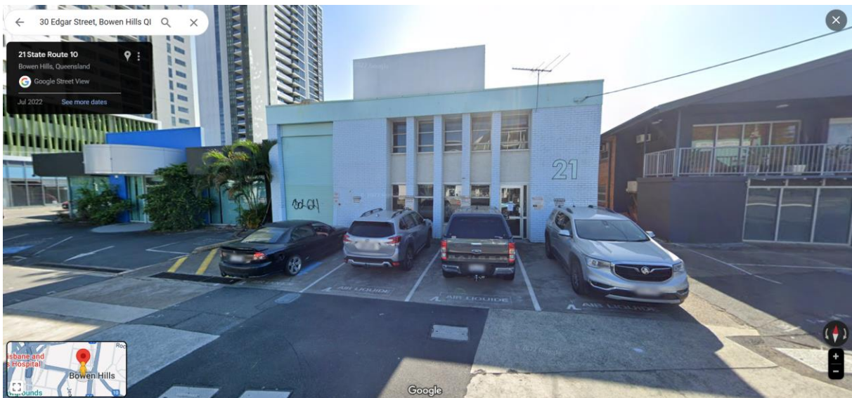
Figure 2-10 21 Campbell Street, Bowen Hills Source: Google Maps
