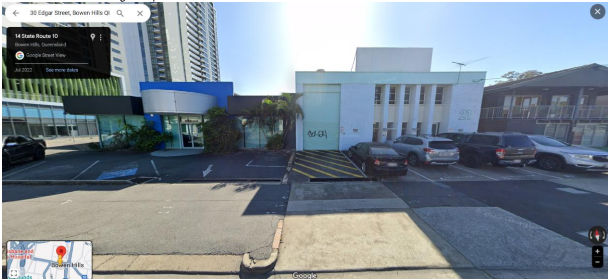
Figure 2-9 21 Campbell Street, Bowen Hills Source: Google Maps
