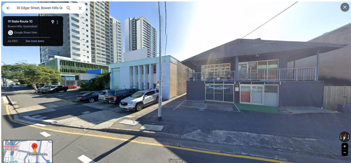
Figure 2-12 19-21 Campbell Street, Bowen Hills Source: Google Maps
