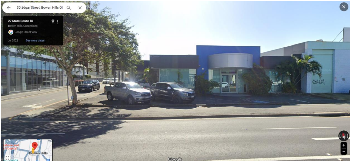
Figure 2-8 25-27 Campbell Street, Bowen Hills Source: Google Maps
