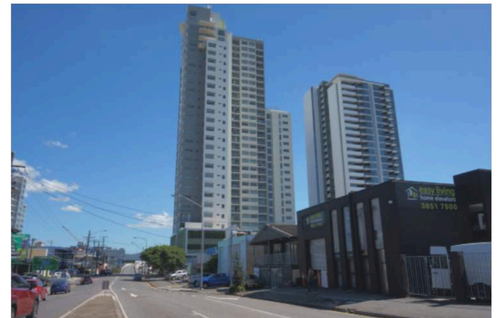
C Campbell Street
