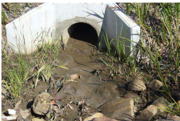
Figure 17 Sediment accumulated at an inlet
