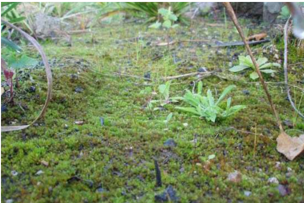
Figure 23 Moss growing on the filter bed surface
