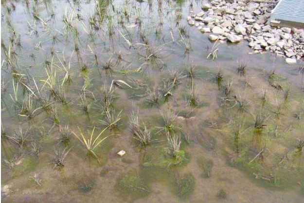
Figure 22 Algae growing on the filter media surface
