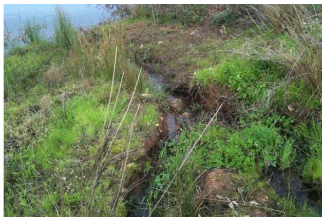
Figure 15 Erosion at the transition between wetland cells
