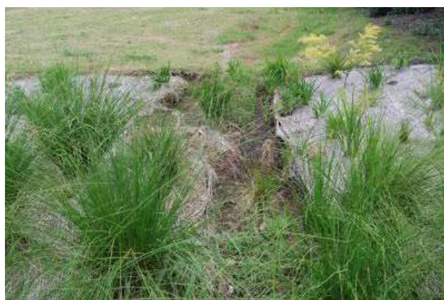
Figure 15 Erosion at the transition between wetland cells
