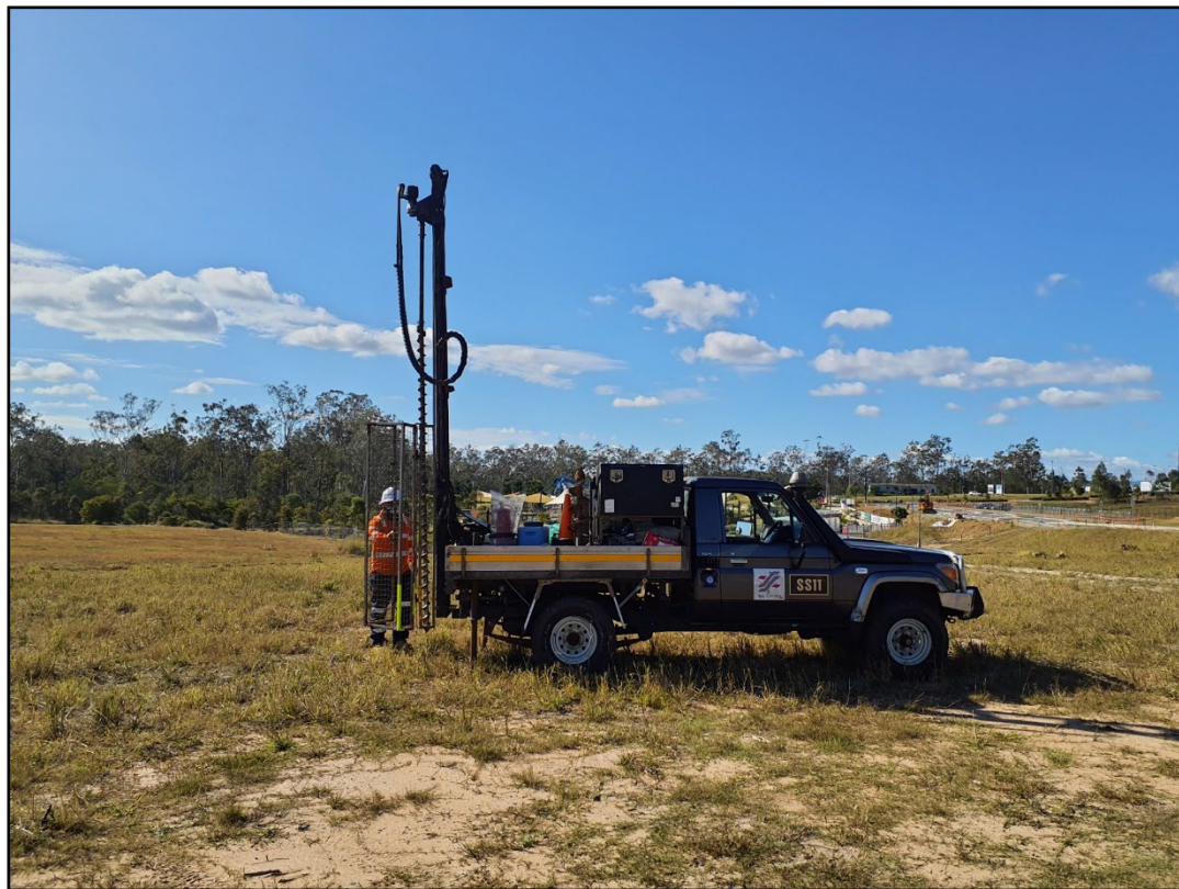
PHOTOGRAPH 1 – BH01 LOCATION, FACING EAST ACROSS THE SITE
