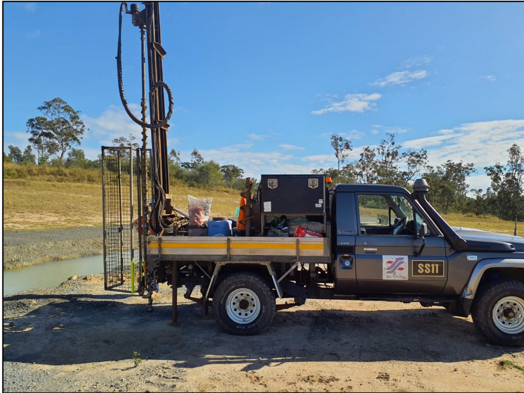
PHOTOGRAPH 2 – BH02 LOCATION, FACING NORTH INTO THE SITE
