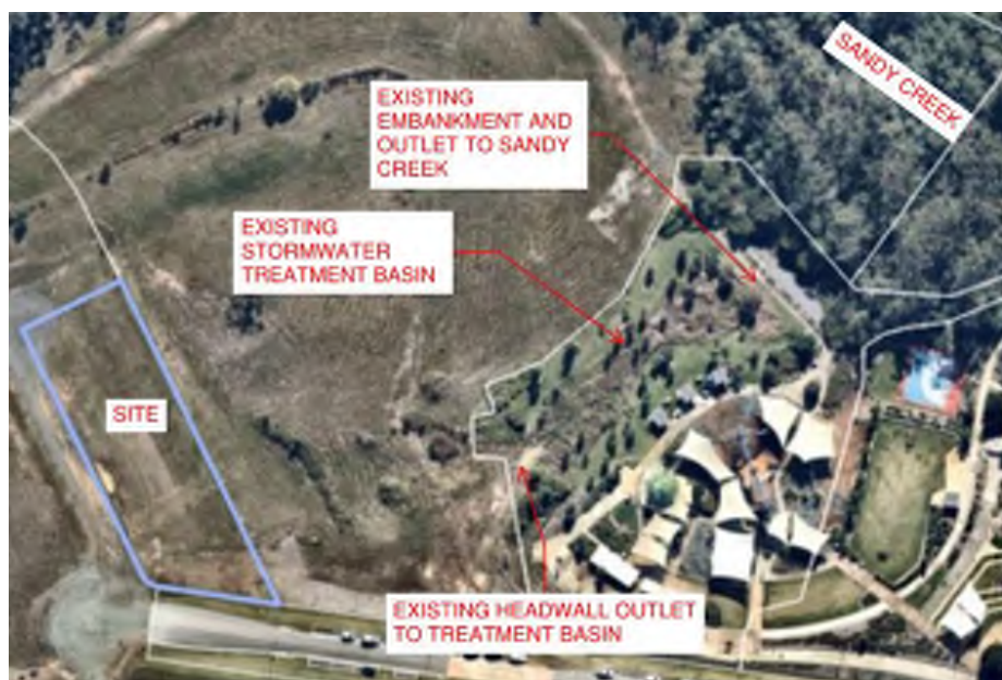
Figure 7 Aerial Imagery of constructed stormwater treatment basin (Nearmap)
