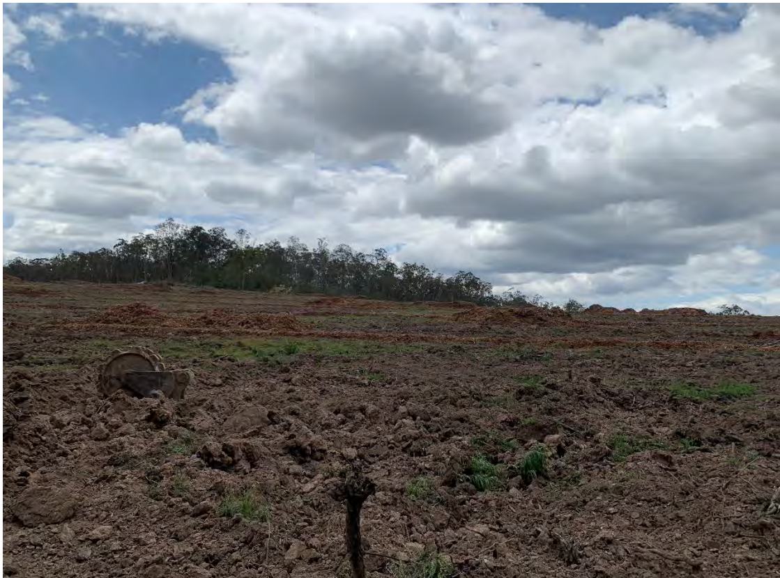
Plate 6 – Gentle sloping terrain in the central portion of site on northern side of main drainage channel near test pit TP21 which has been stripped and tyned.
