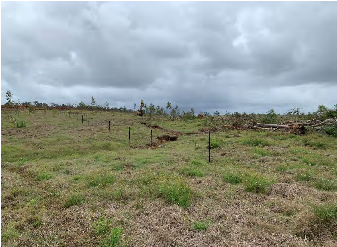
Plate 11– Erosion within drainage feature within north eastern portion of the site.
