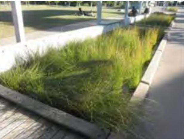
Example of Rain Gardens
