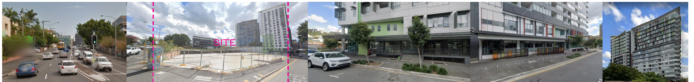
Water Street - North Elevation
