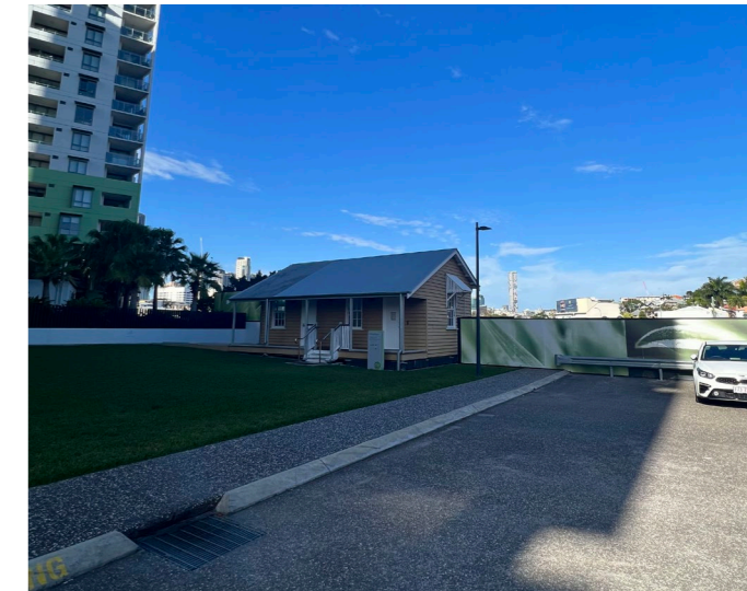
12 Facing south west towards the Orderly Room, a Local Heritage listed building
