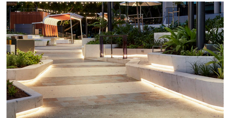
Strip lighting recessed into walls & bench seats to highlight nodes
