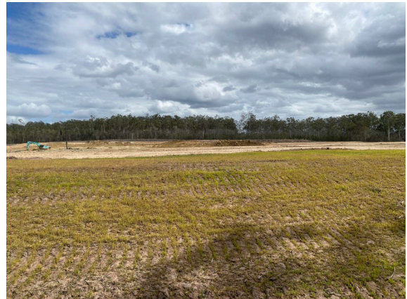
Photograph 3.6 Future wetland and stormwater management structures at F
