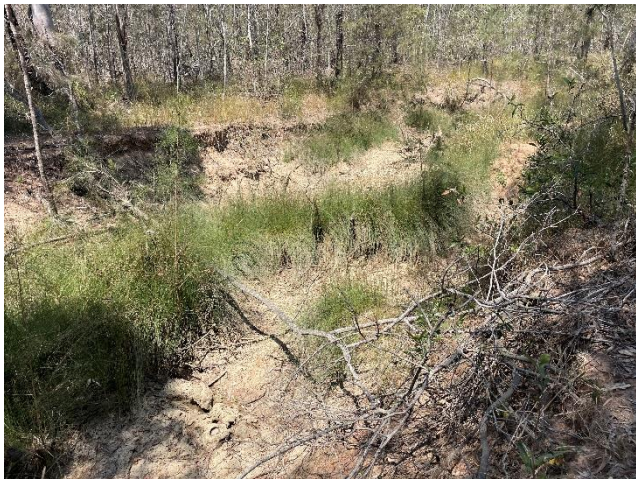
Location 7 – Waterway Widened with Exposed Banks
