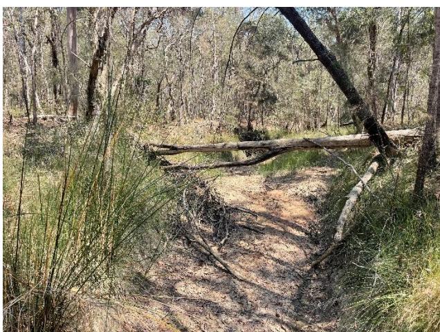
Location 11 – Bank Erosion and Split Waterway
