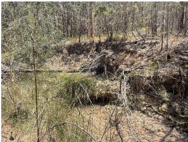
Location 9 – Bank Erosion to Outside Bend
