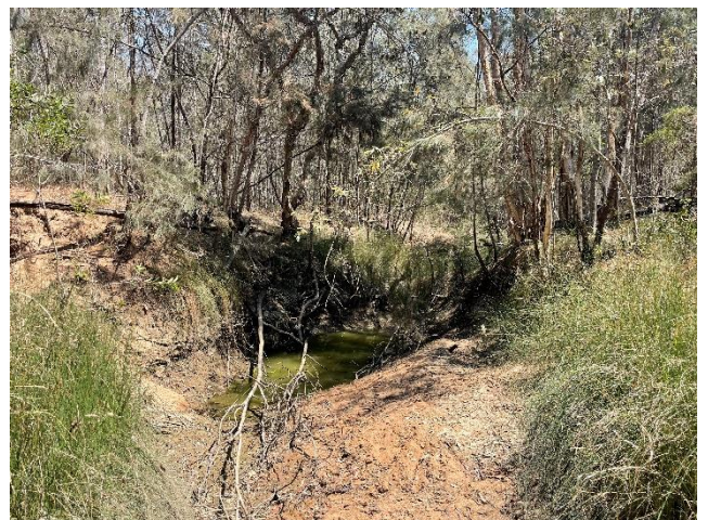
Location 10 – Headcut Location 1
