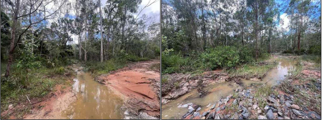
Photo Set 3: Drainage features present within Precinct 5 & 6
