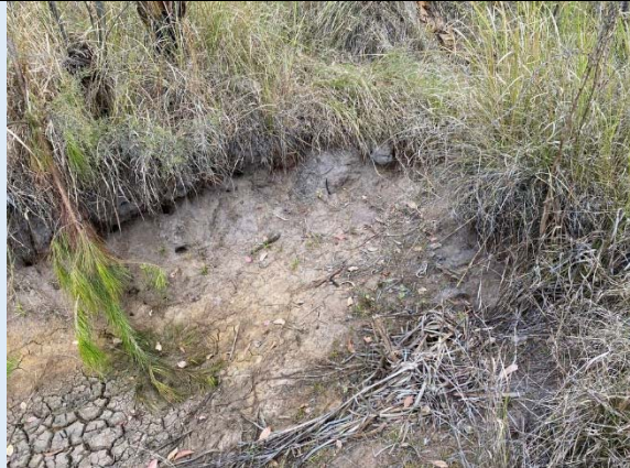
CH0-50 Low flow channel evident with isolated scour pool (dry) approx. 10m long, 3m wide surrounded by dense groundcover vegetation. Fill, provide rock lining and interplant with grasses/shrubs. Will likely form part of road crossing works.
