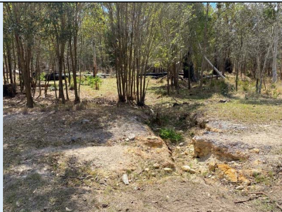
CH1000-1120 Shallow low flow channel commences and extends upstream with gradual deepening and evidence of scour. Fallen logs increase scour locally (while still shallow). Surrounding area broad, flat and well grassed. Vehicle track crossing at CH1120 with localised washout of gravel. Local filling with non-dispersive soil and revegetation. Monitor stability and natural regeneration of vegetation surrounding. Where continued instability occurs in low flow, local rock scour protection may be required.
