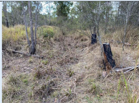
CH50-100 Low flow channel evident with emergent wetland plants (now dry and died back). Surrounding area densely vegetated with grasses/shrubs. Monitor area as development progresses to assess resilience. No obvious instability at present.
