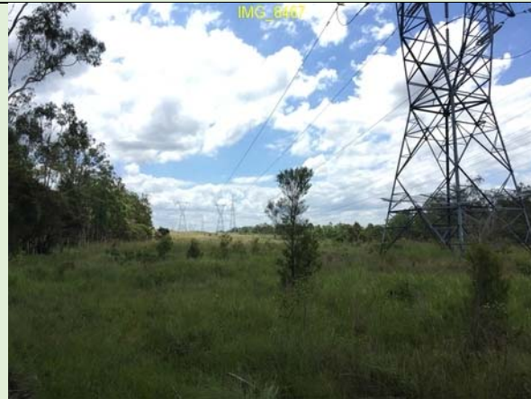
CH0-200 Powerline easement is fully cleared (grasses and some immature regrowth remain), broad flat scattered boggy zones.
