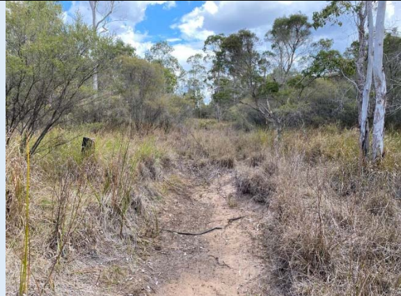
CH0-50 Low flow channel evident with isolated scour pool (dry) approx. 10m long, 3m wide surrounded by dense groundcover vegetation. Fill, provide rock lining and interplant with grasses/shrubs. Will likely form part of road crossing works.
