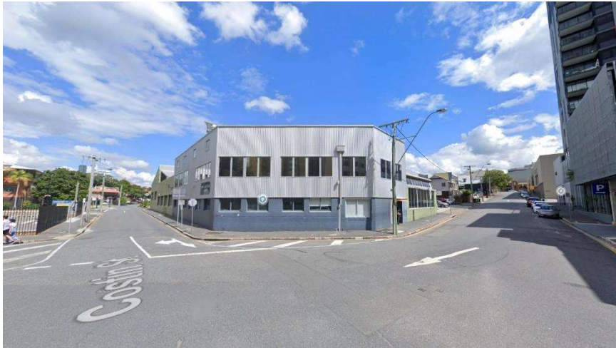
Figure 1: Site Frontage (Source: Google Street View)
