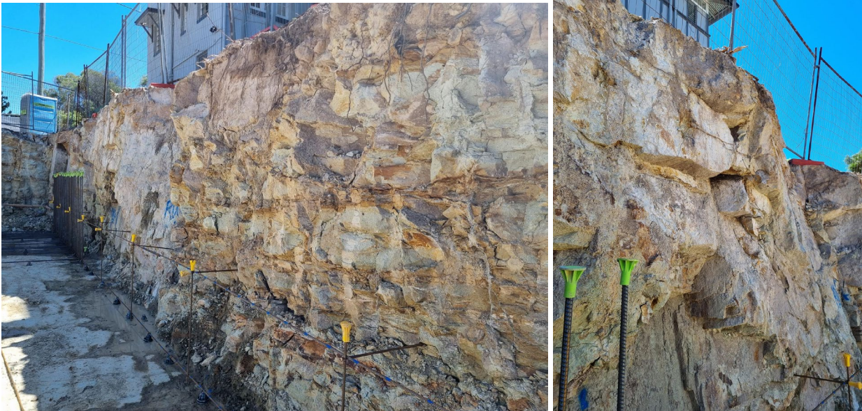
Images 10a and 10b – Nearby excavation face in Tuff (St Pauls Terrace)
