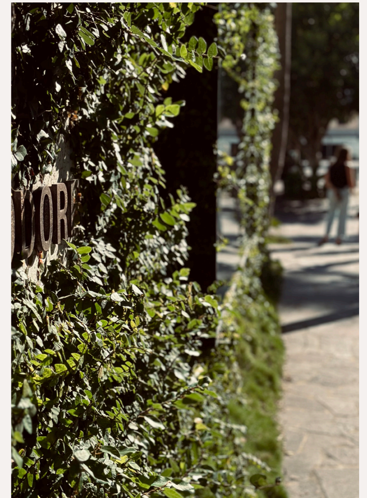
Climbers to create vertical greenery on walls to balance built form with landscape
