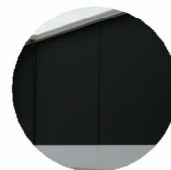
CONC-02/03/04 Painted Concrete Tilt Panel Wall
