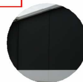
CONC-02/03/04 Painted Concrete Tilt Panel Wall
