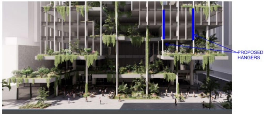
Figure 36 - Hanging Structure to Podium
