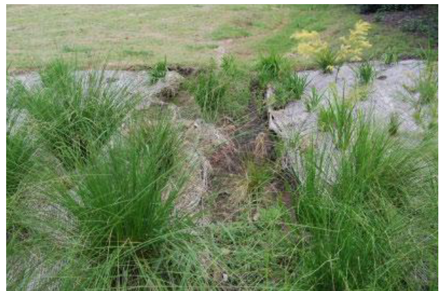
Figure 15 Erosion at the transition between wetland cells
