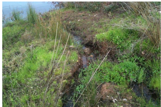
Figure 15 Erosion at the transition between wetland cells
