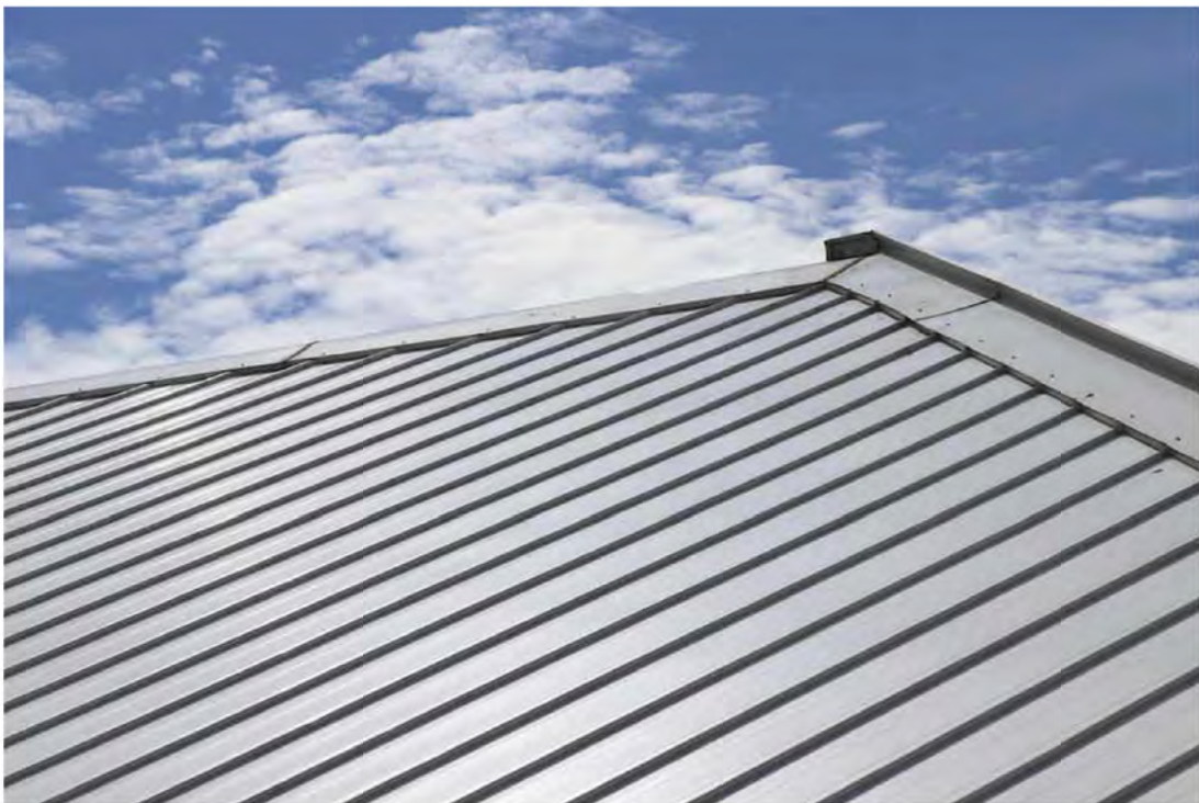
4. PROFILED METAL ROOFING
