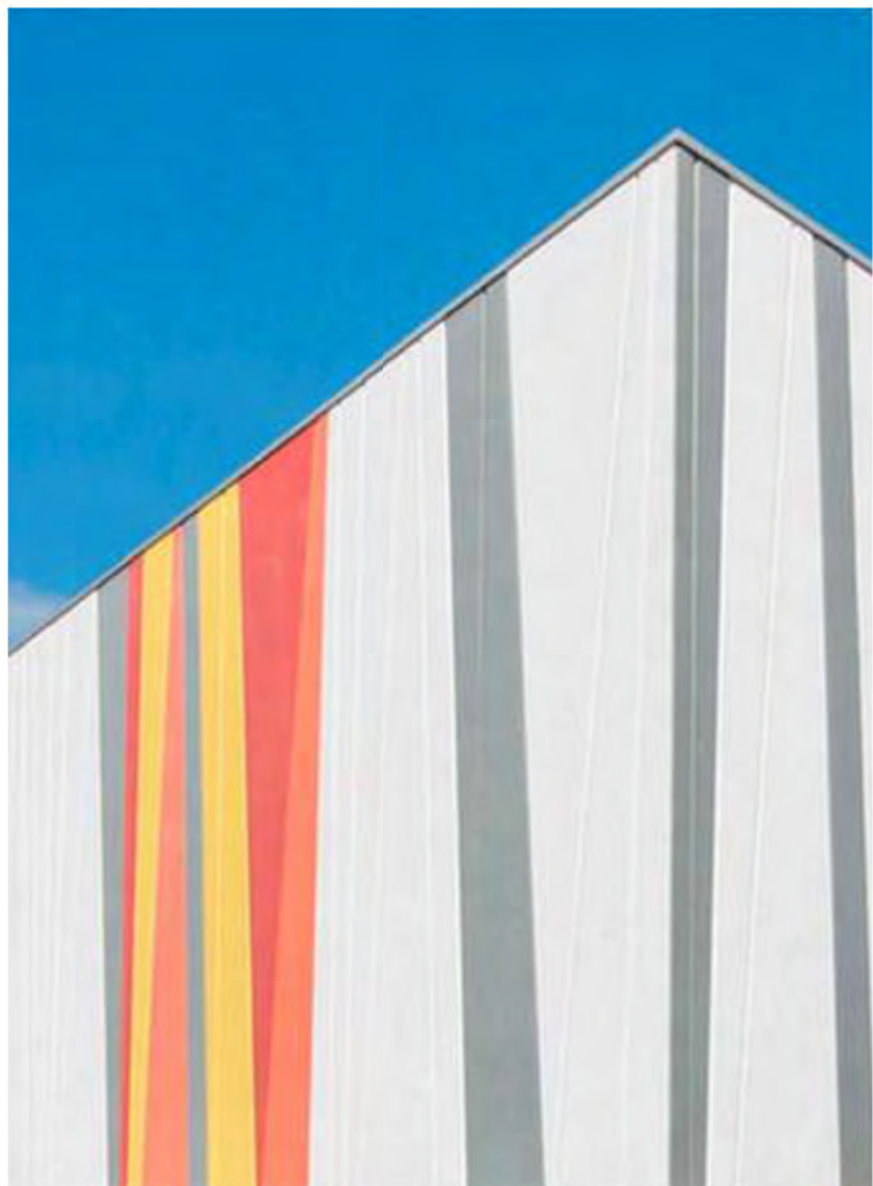
7. PAINT FINISH CONCRETE TILT-UP PANELS
