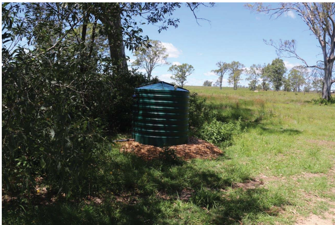
Photographic Plate 8: Potable water storage for each cabin is located within 100m of the cabin site and is not used for firefighting purposes.
