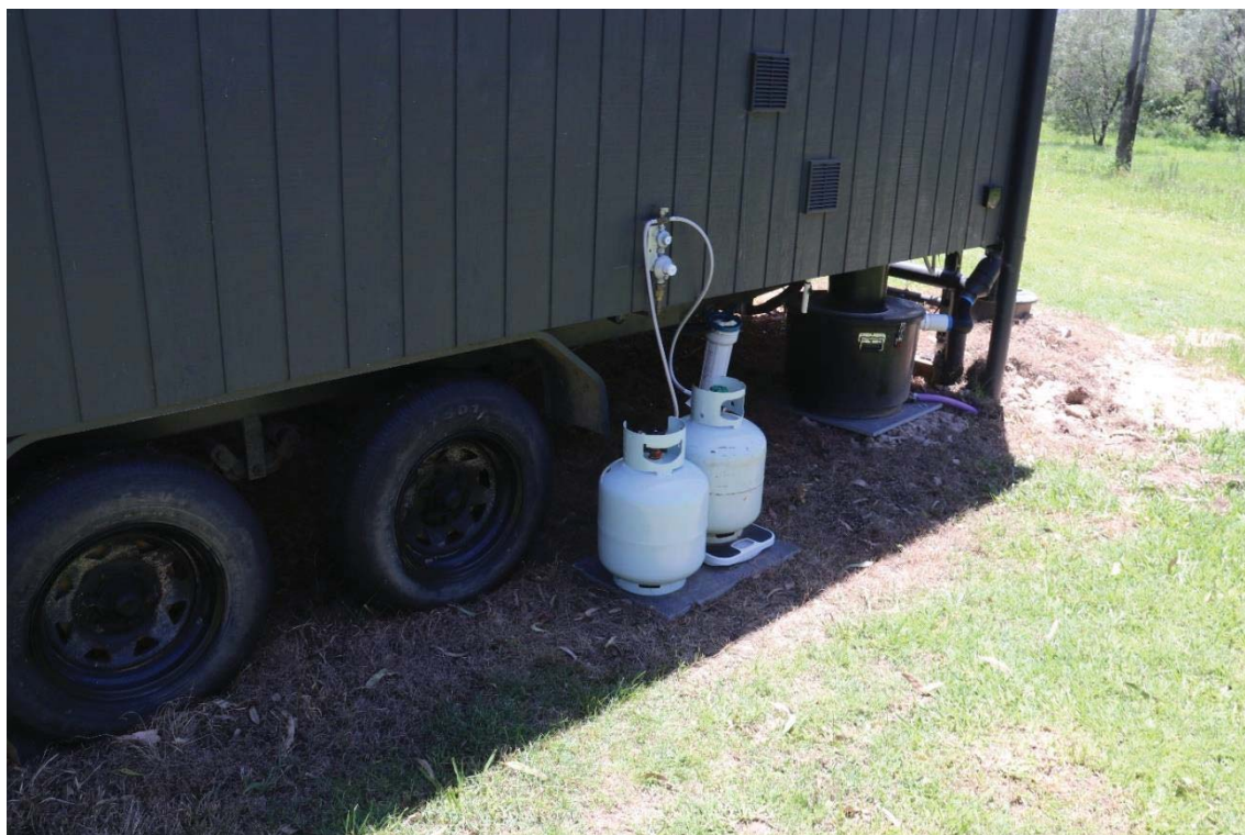
Photographic Plate 9: Gas tank storage is located on a concrete slab at each location. Weed and vegetation control is undertaken under the cabins and around the gas storage areas.
