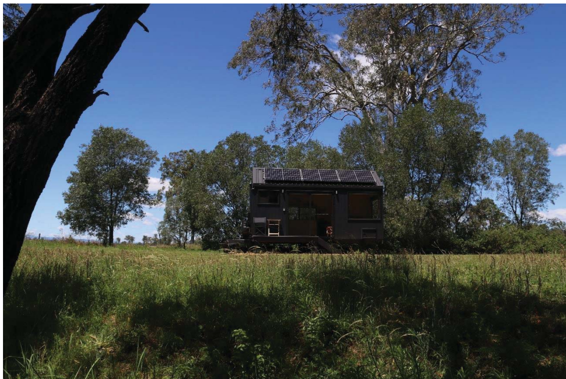
Photographic Plate 1: View of Cabin Cybele from the creek bank to the north of the location. The grass up to 10m from the cabin and campfire area is maintained at 100mm. Pasture areas greater than 10m away are regularly slashed or grazed
