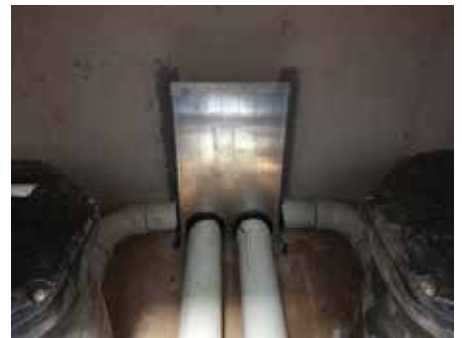
Figure 3 - Typical Outlet Weir Wall
